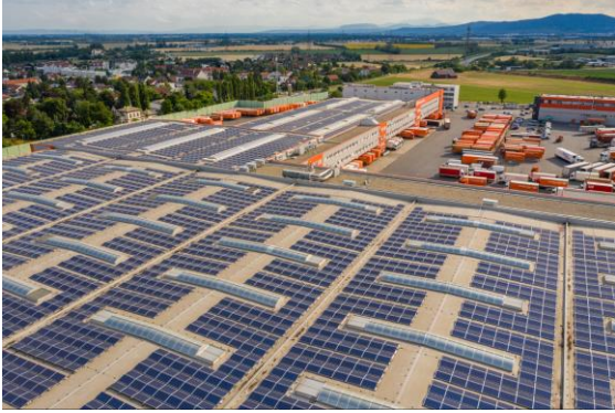
CAPTION: Around 2.4 million kilowatt hours of electricity every year are generated over an area of approximately 21,500 square meters. (Source: Ursprunger / Media Solutions)
