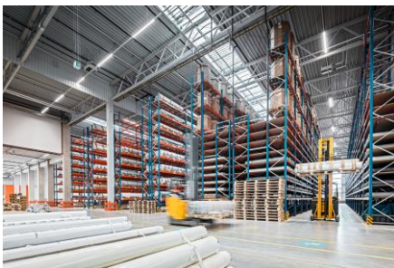
Caption: The site comprises a 16,500-square-meter logistics hall and a handling area of 6,500 square meters. (Source: Gebrüder Weiss / Wolfgang Croce)
