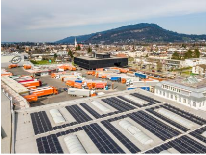
Caption: Gebrüder Weiss will save around 1,050 tons of CO 2 annually with solar power installations by the end of 2021. Here: the new photovoltaic system at the Lauterach / Austria location produces 440 megawatt hours (MWh) of electricity per year. (Source: Gebrüder Weiss / Sams)
