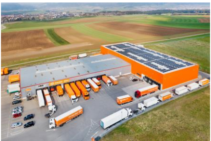
Caption: The solar power installation at the Gebrüder Weiss location in Aldingen produces 280 megawatt hours (MWh) of electricity per year (source: Gebrüder Weiss / Matt Stark)
