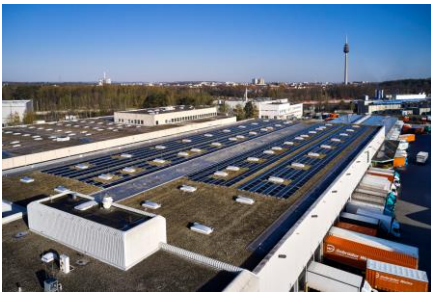
Caption: The solar power installation at the Gebrüder Weiss location in Nuremberg produces 540 megawatt hours (MWh) of electricity per year (source: Gebrüder Weiss / Tilman Weishart)
