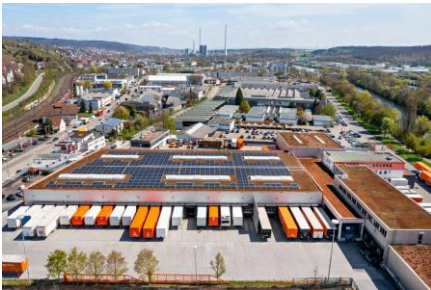
Caption: Gebrüder Weiss produces 280 megawatt hours (MWh) of solar power per year at its Esslingen location (source: Gebrüder Weiss / Matt Stark)
