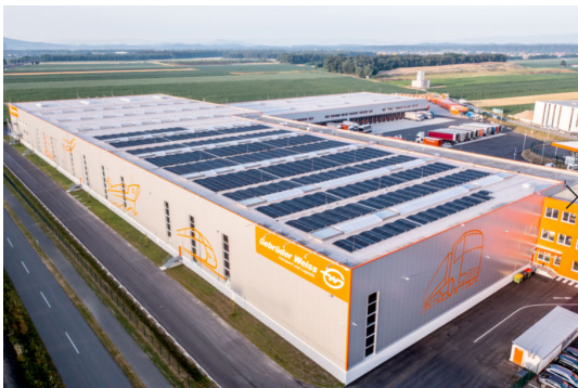
Caption: The new Gebrüder Weiss photovoltaic system at the Graz location. (Source: Gebrüder Weiss / Art-Media)
