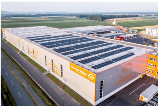
Caption: A criterion for gold certification: the photovoltaics plant at the Gebrüder Weiss location in Graz produces electricity in the amount of some 460 megawatt hours – enough to meet around half of the energy needs of the 27,000 square meter logistics center. (Source: Gebrüder Weiss / Art-Media)
